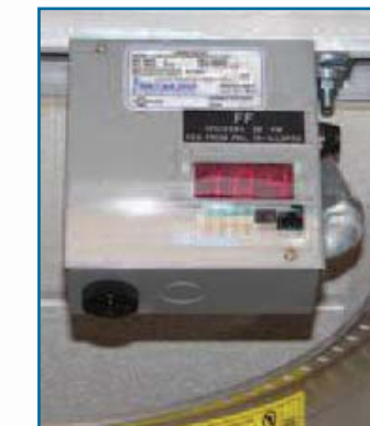
Power monitoring is available to measure phase loads, provide alarm functions, onboard LED displays, and/or remote communication of information. Monitoring can be built into the power feed unit (redundant runs shown) or as a plug-in monitor (right).
