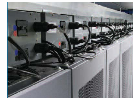
Plug-in units are offered with a wide variety of receptacles, circuit breakers, and drop cords. Multiple circuit breaker plug-ins are offered and can be used in high-density applications.
