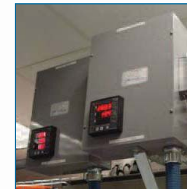
Power monitoring is available to measure phase loads, provide alarm functions, onboard LED displays, and/or remote communication of information. Monitoring can be built into the power feed unit (redundant runs shown) or as a plug-in monitor (right).
